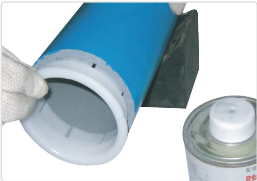
▲ Application of anti-corrosion sealant and insertion of a pipe end protection ring
